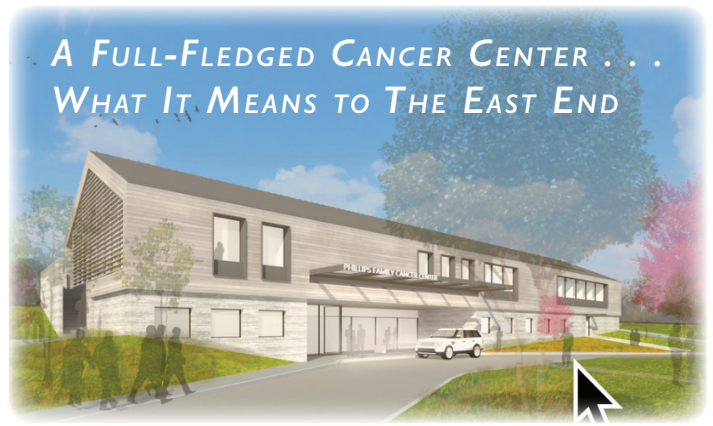
Architect's Rendering of the New Southampton Cancer Center (located on Route 27 across from Storms Ford Dealership).
